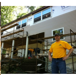
Steve replacing siding
